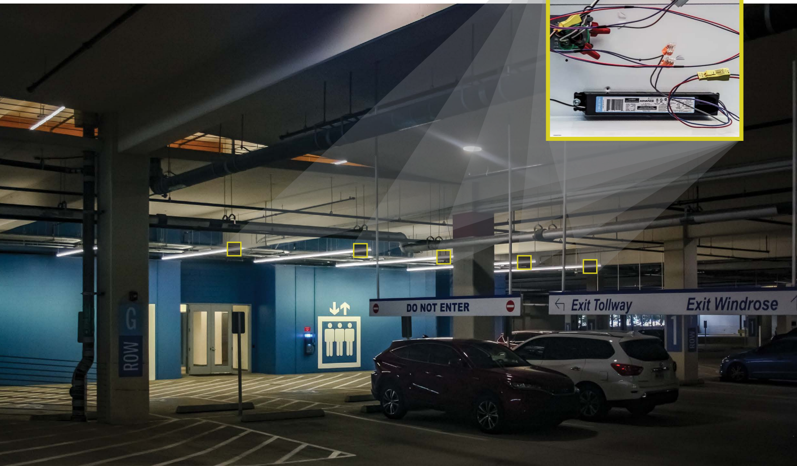
Detail of Casambi node retrofitted into every fixture.
